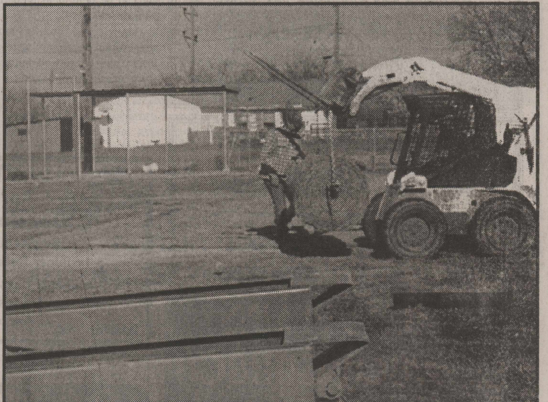
LAYING THE SOD—men working in the sunshine on Friday putting down the new grass
