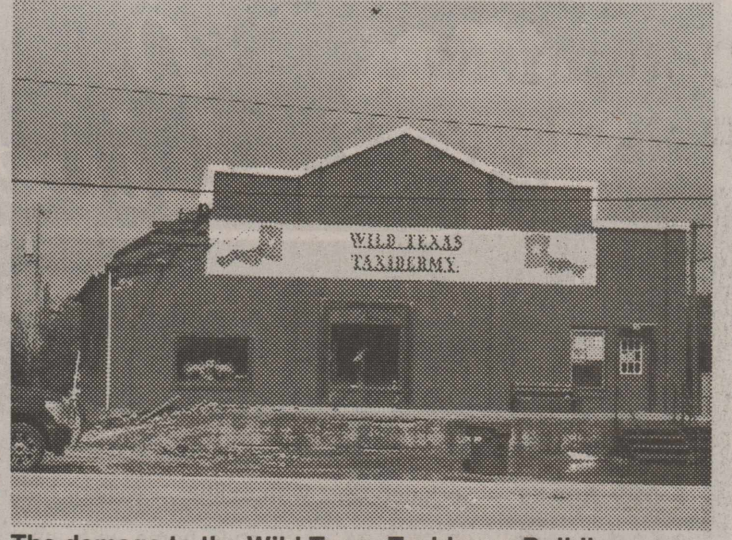
The damage to the Wild Texas Taxidermy Building.
