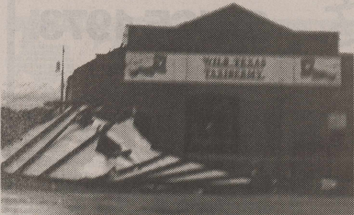
Part of Subway's roof landed on the Wild West Taxidermy Building.
