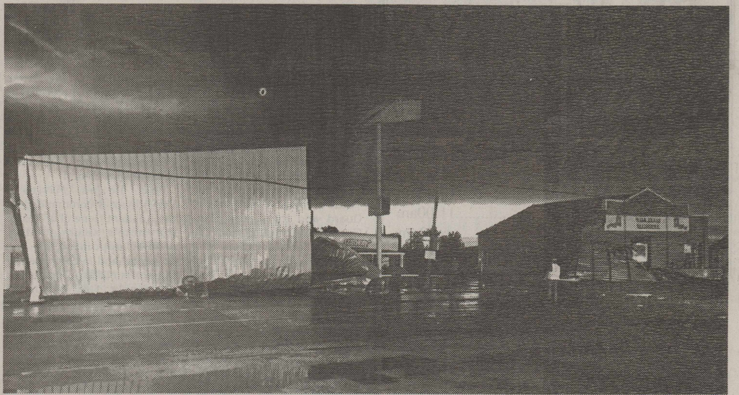
Storm Damage at Subway and Wild Texas Taxidermy. Photo taken right after the storm came through.
