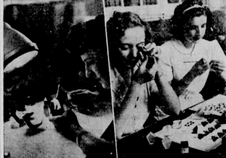
The girl at left is cleaning optical elements that will later be assembled into a battery commander's telescope. Right: Two pretty maids check on finished prisms and lenses.
