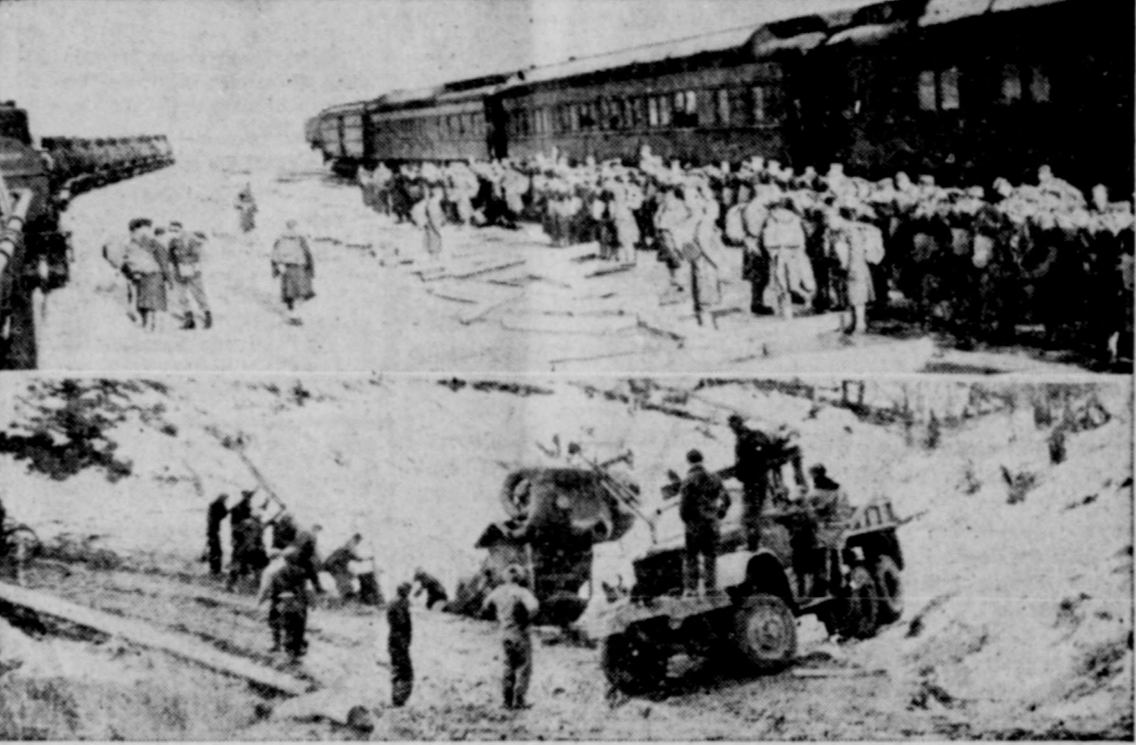
Upper picture shows journey's end, as U. S. engineer corps troops arrive at the end of the steel ribbon, at Dawson Creek, B. C., to start building a highway to Alaska from the end of the present road at Fort St. John. Below: First activity of road building at start of construction of the Alaska highway. Note men in foreground with truck pulling another road-building truck out of a ditch. All equipment for the project was shipped from the States.
