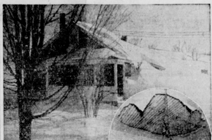
When gutters and downspouts are clogged, melting snow and ice back up under shingles. Seeping into the interior, the moisture cracks plaster, stains wallpaper and rots the structure. A light roof is the first fundamental of sound shelter.
