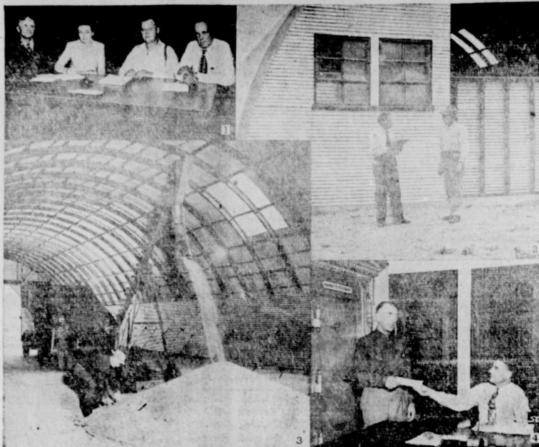
One of the Nation's first farmers to purchase new crop storage facilities through the CCC financing program is Irvin McKibben of Maddock, N. D. Steps by which he completed the transaction form a pattern of experiences which will be shared by thousands of wheat and corn growers this Summer and Fall as their own applications are processed. They are shown in the photo-story above.
