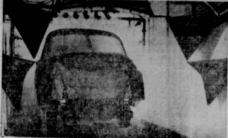
Newest test developed by Fisher Body is this "water bath" in which hundreds of gallons of water are shot at each body. An inspector rides inside the body through the test, searching for a possible leak. The rubber shroud covering the dash panel prevents water from entering holes there for the steering wheel, pedals and for the wiring.
