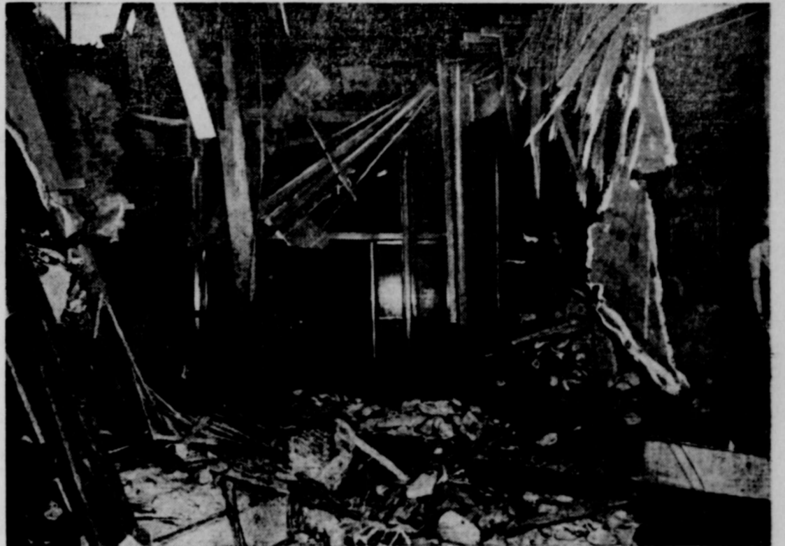
SHOPPERS TRAPPED AND KILLED . . . Two persons were killed and many others were trapped by falling beams and ceiling when the roof of this building, a Lerner's clothing store, collapsed. The tragedy took place during the violent earthquakes that rocked Bakersfield, Calif. The building is typical of the damage done to stores in the downtown area of the California city. However, other shoppers in the downtown area were fortunate that some of the roofs resisted the quake and remained secure, as it was this type of damage that caused most of the deaths reported after the Bakersfield quakes. Scientists foresee a year more of California quakes.
