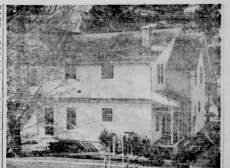
This 60-year-old farmhouse has been remodeled into two apartments. Outside stairs to the second-floor apartment can be seen at the left in the close-up view above. The overall view, right, shows the house as it stands in the Wisconsin countryside. Sidewalls are painted white, and heather-colored asphalt shingles cover the roof.
