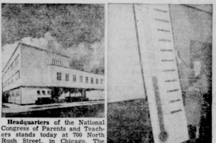
Headquarters of the National Congress of Parents and Teachers stands today at 700 North Rush Street, in Chicago. The building, dedicated in 1955, won an award from the Chicago chapter of the American Institute of Architects and the Chicago Association of Commerce and Industry for excellence in architecture.
