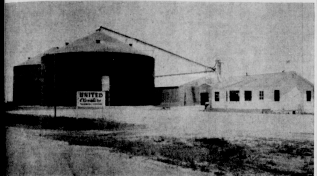
PICTURED ARE THE new grain storage tanks which have been recently completed at the Silverton branch of United Elevators. At Claytonville one of these units is now under construction. Each of these conical steel buildings will house half a million bushels of grain. Farris Martin, manager of the Silverton Elevators, reports that most of the barley in Briscoe County has been harvested. He states
