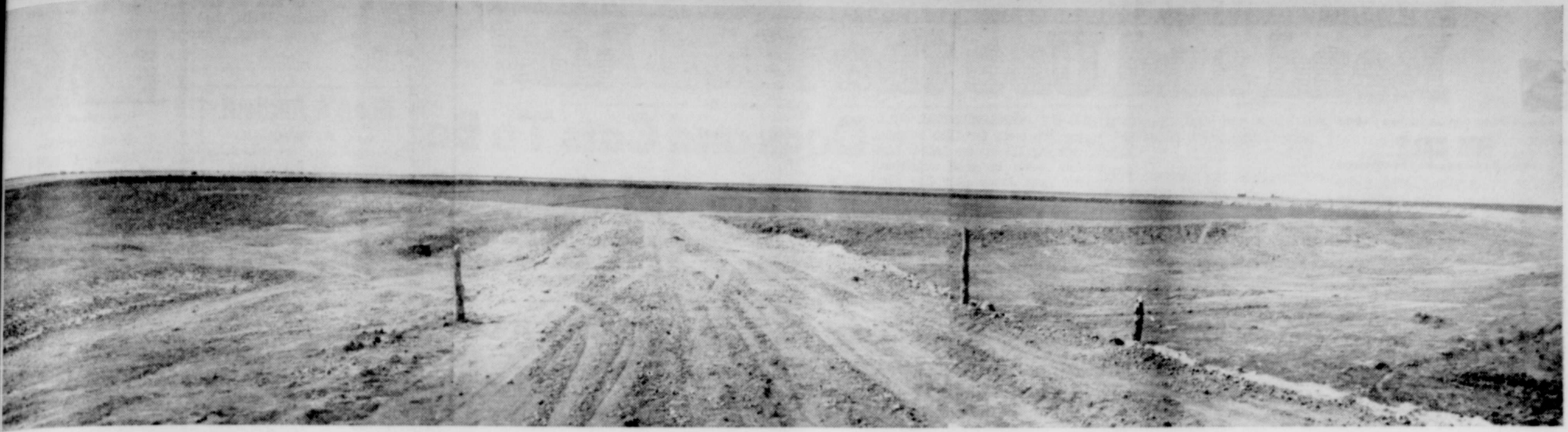
A PANORAMIC view of the dike with cattle grazing peacefully in the distance is seen looking west. The Elton Cantwell
