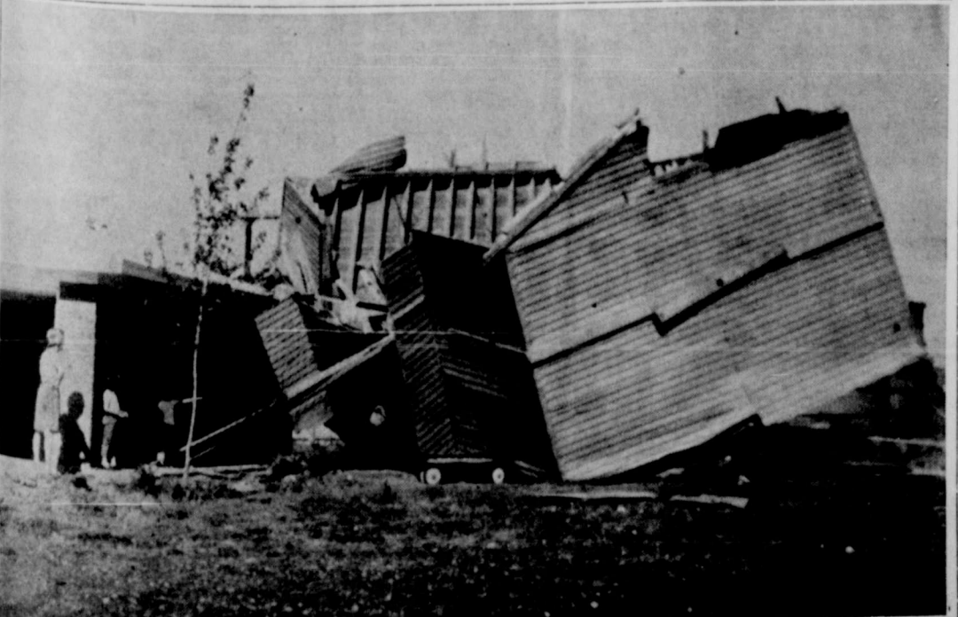
The home of Mr. and Mrs. Norman Strange was damaged when a granary was lifted off its foundation and dumped over in their yard. A small metal grain bin was also blown into the twisted mass which had been the granary. —Briscoe County News Photo
