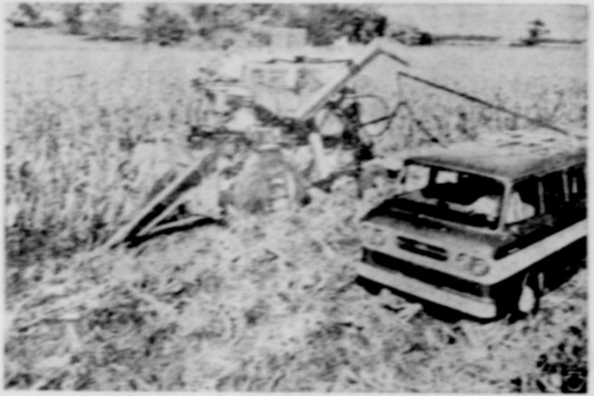
A mobile laboratory crammed with gear "electrocardiographs" a Gleaner combine working in an Indiana cornfield. Delicate electronic fingers take the "pulse" of the machine. Complex circuitry records the amount of power required to run fans, elevators and other parts.
