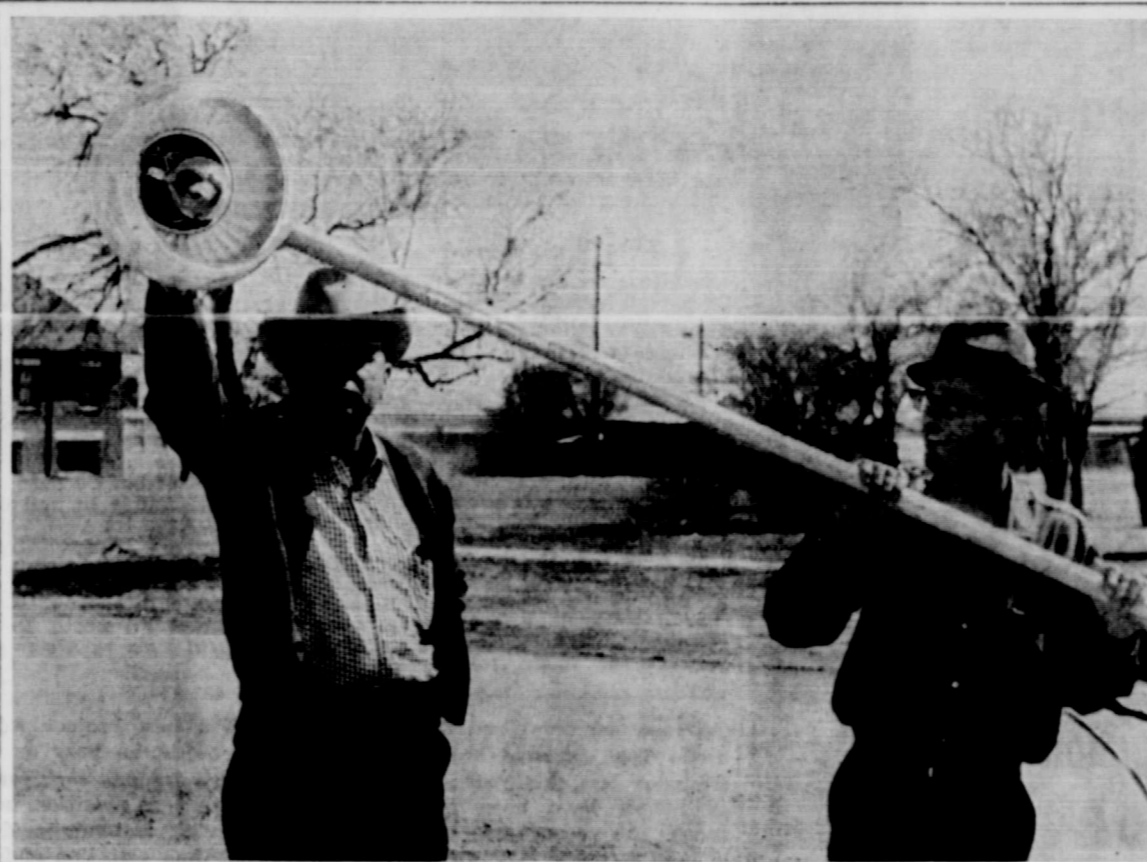
Mayor Jimmie House and Kenneth Tate, are being installed here. Twenty-six new manager of Southwestern Public Service street lights are being put into service and Company in Silverton are shown inspecting 34 old street lights are being converted to one of the new mercury vapor lamps that mercury vapor. (Briscoe County News Photo)
