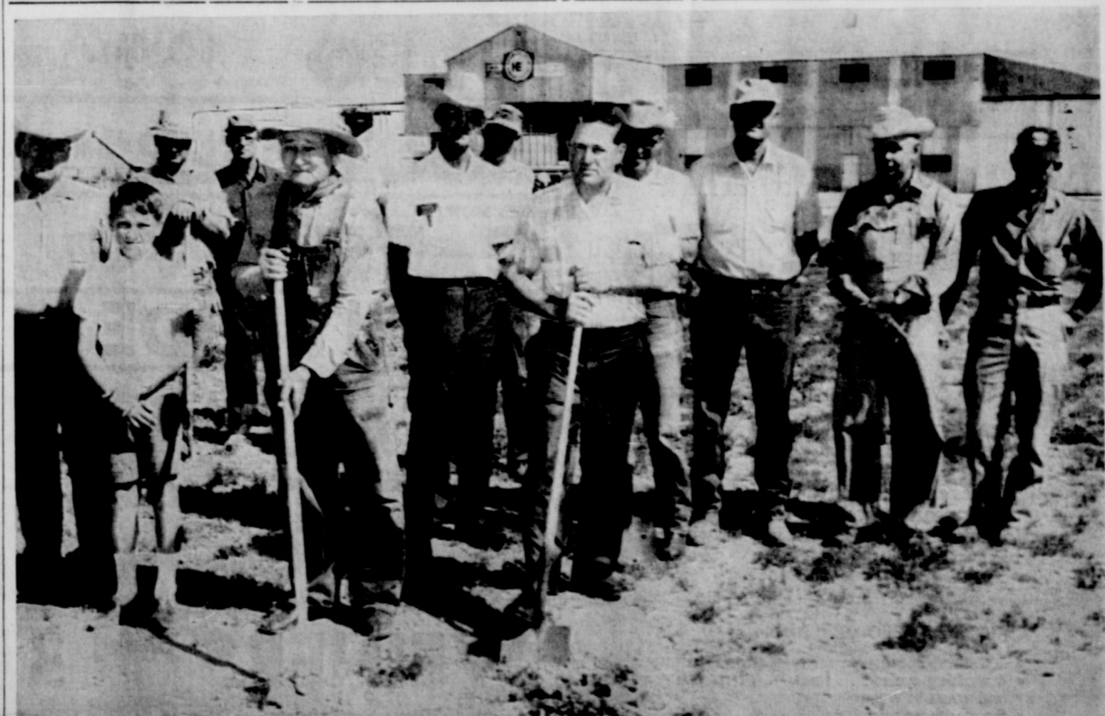
Farris Martin, Micki Jasper, John Francis, J. D. Nance, Carron Garrison, Aubrey Rowell, Edwin Dickerson, Clyde Mercer, Sam Lewis and Kenneth Hooten look on as Louis Francis and Ray Teeple break ground for the new $50,000 elevator leg to be built by Briscoe Co-Op Gin. Plans are to truck the grain to Plainview to Producers Grain Corporation. The ground-breaking ceremony was held Wednesday last week. (Briscoe County News Photo)
