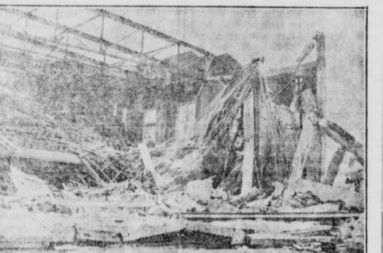
People who have never gone through a tropical hurricane cannot appreciate the ordeal endured by citizens of the Lower Texas valley, nor visualize the destruction of the twisting wind. Above is a picture of the municipal auditorium at Harlingen, showing great masses of concrete twisted and broken. Below the freight docks at McAllen are pictured in splinters.
