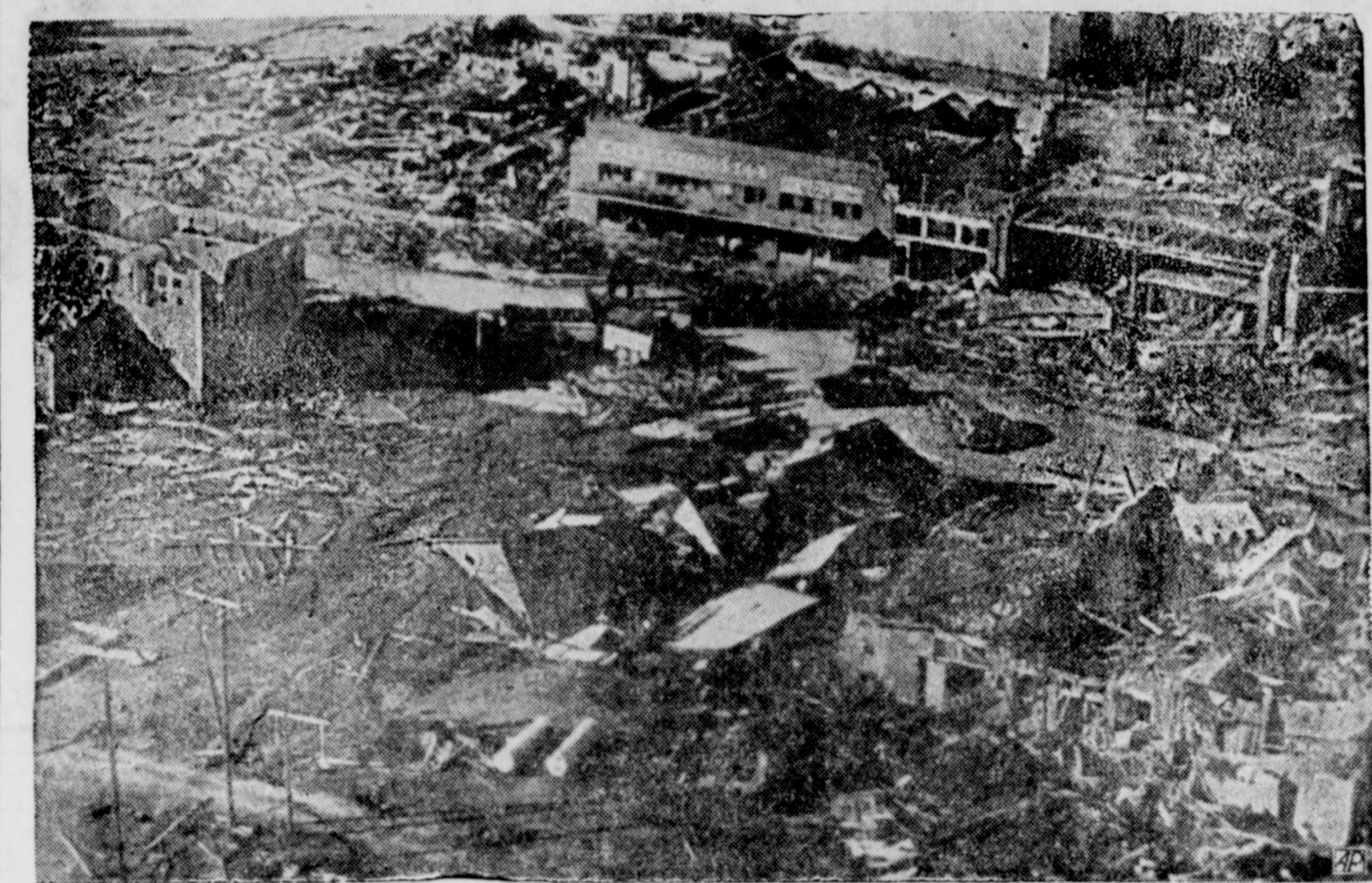
HERE IS A PORTION of the wrecked business district of Higgins, one of several Texas and Oklahoma Panhandle towns struck last Wednesday night by tornado which left death and
