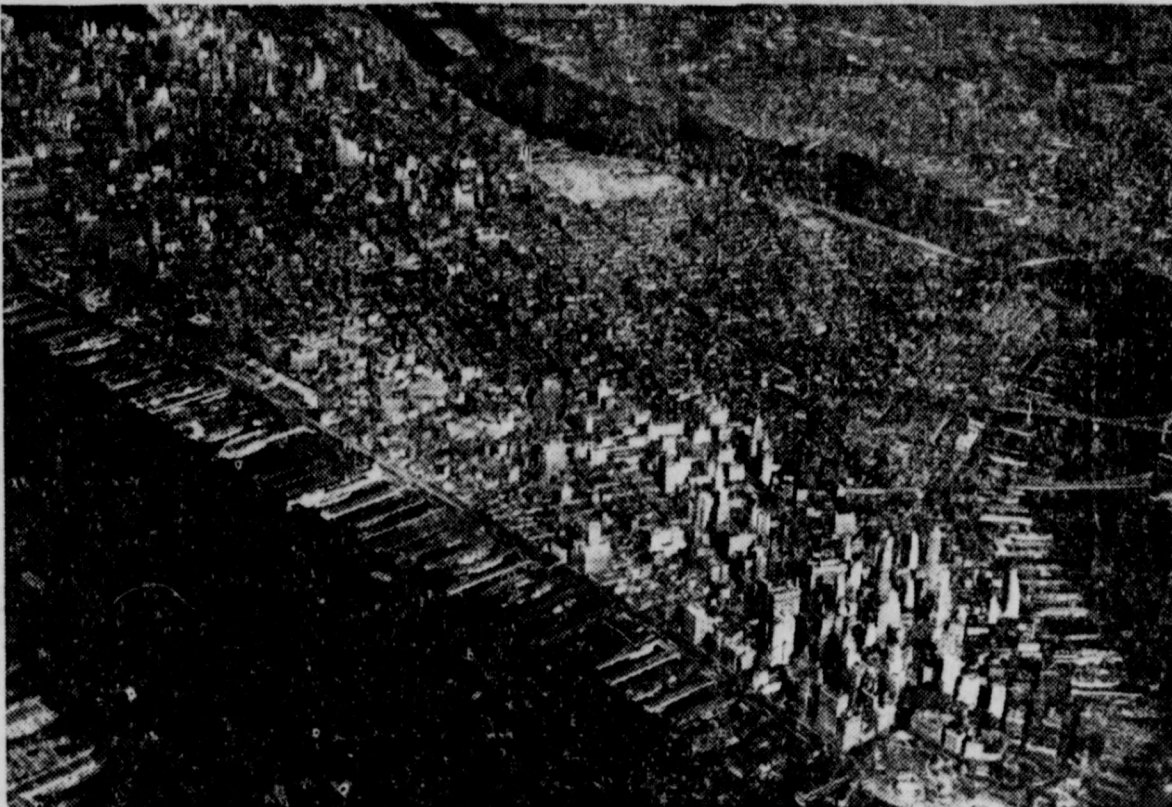
BLANKET OF STEEL . . . In this aerial photo of Manhattan Island, made from an altitude of 7,500 feet, can be seen the greatest concentration of steel to be found anywhere in the world. Some 27 million tons of it went into the building of skyscrapers, bridges, subways, docks and other facilities that go to make up a great city. Steelways magazine points out that to duplicate that amount of steel would require enough iron ore to cover Manhattan's 22 square miles with a nine-inch blanket.
