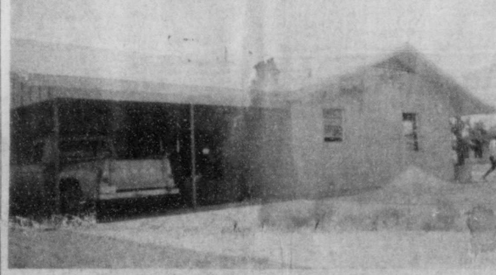
South entrance. 2 car-carport.
