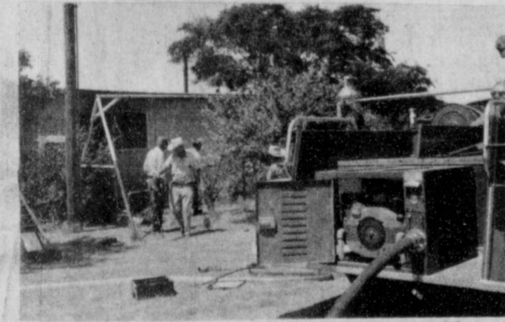
Top picture show some of exterior damage at T. M. Randolph home Tuesday. Bottom picture is Roby Firemen battling the blaze.
