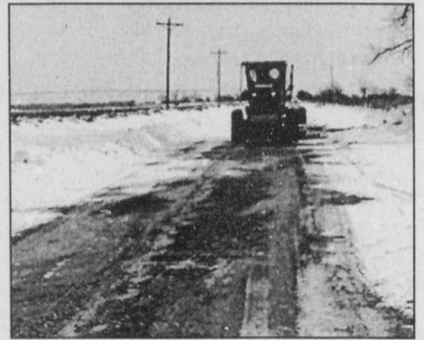
A county blade scrapes foot-deep snow off a 1-mile section of County Road 1018 where bare fields allowed snow to drift.
