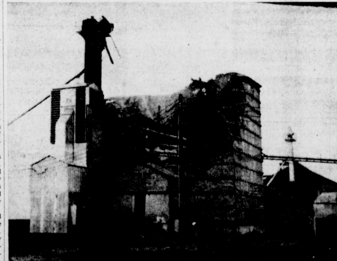
$164,000 BLAZE — Here's the Earth Elevator after a $164,000 fire swept the main structure Thursday morning. Firemen from five towns fought the blaze for 2 1/2 hours before bringing it under control. (Journal Photo & Engraving)
