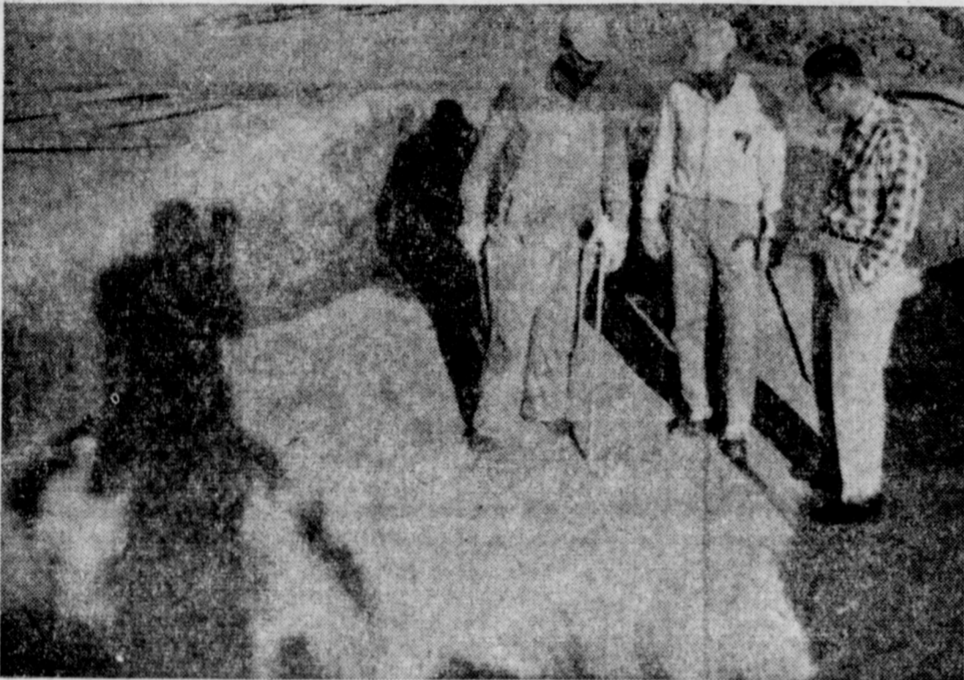
FALLOUT SHELTER — Here's probably Bailey county's first fall-out shelter being built on the W. E. (Dick) Chisholm farm at Needmore. The shelter is located behind a new two-bedroom brick home under construction also. Walls are eight inches thick and the roof has 10 inches of dirt. The project is financed by the Farmer Home Administration. The pictures above show forms being removed from inside the 10 by 12-foot shelter, and the concrete top of the shelter (before dirt is placed on top, and the entrance way. With the picture are Chisholm and a helper and John C. Kennedy, county FHA supervisor. (Journal photos and engravings)
