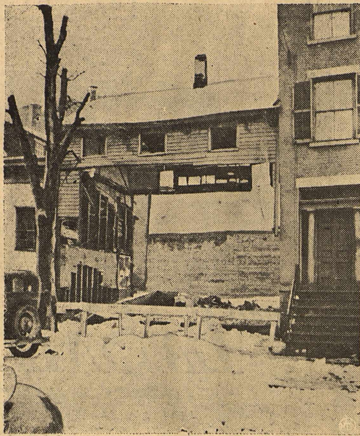
Some one stole two floors of the Albany, N. Y., house not shown above. When last seen they occupied the space directly above the attic—all that remains of the wooden home. Police investigating this unusual theft believe the house was taken apart piece by piece and carried away for fuel during recent cold snap.
