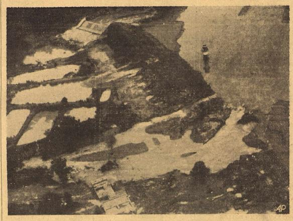
A section of the Cleveland, Okla., dam which was washed out with an estimated damage of \$50,000 caused by flash floods in northeast Oklahoma, is shown above in this air view. In the lower center is the foundation of the city powerhouse, carried away by the first surge of water.
