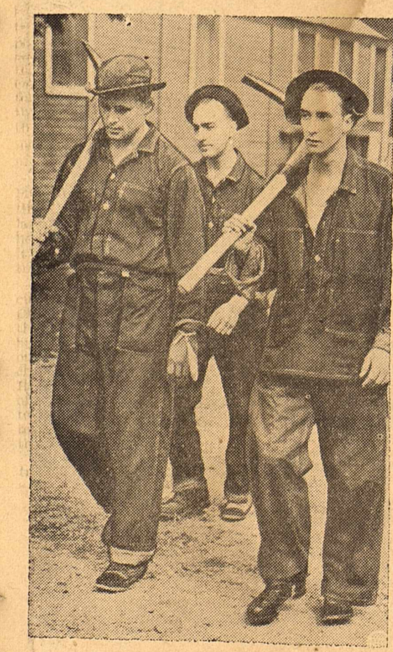
Pvt. Sullivan gets a different taste of Army... when a day of fitting, drill, and labor is over, life. At right, above, with fellows members of the Pvt. Sullivan is ready for a bit of relaxation. Above, 104th Engineers New Jersey National Guard, he setshe and his pal, Lloyd Roper, also from Chatham, out for a physical labor detail. And... N. J., look over the available movies.
