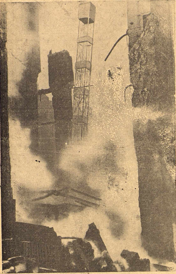
As Nazis poured bombs on London, strange freak left this steel elevator shaft, though listing, still intact, although nearby buildings were demolished.
