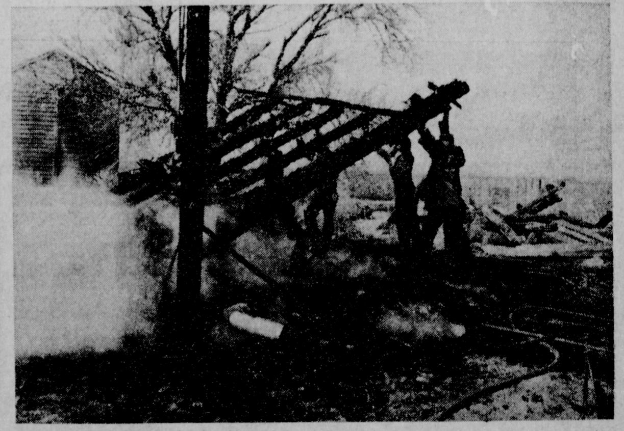
FIRE — Flames completely destroyed a small storage house on the Wiley Barker farm north of Progress this week. Although the fire was battled by two units of the Muleshoe Volunteer Fire Department, the flames had too good a start to bring under control. The small storage place was completely destroyed as were its contents of tools and small items of farm equipment. The loss was estimated at $1,500.
