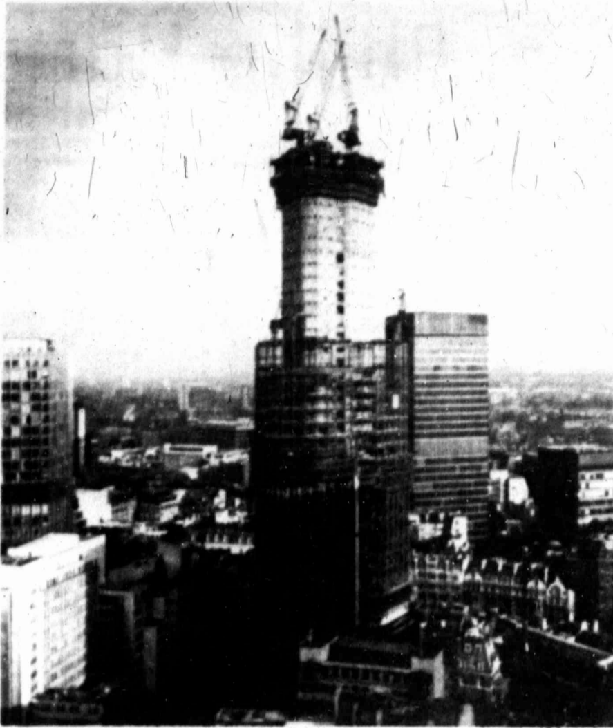
THE NEW TOWER of London rises out of downtown London like a rocket heading toward outer space. The 600-foot structure dwarfs surrounding buildings during construction and is scheduled for completion in 1978.
