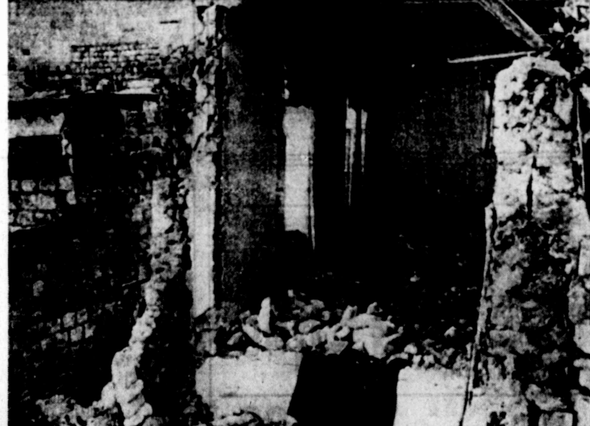
JERUSALEM BOMB BLAST—The wall of a home in the Christian quarter of the old walled city of Jerusalem is reduced to rubble Sunday after a bomb blast tore through the building. Two teenagers were reported killed and five persons were hurt in the blast. (AP Laserphoto)
