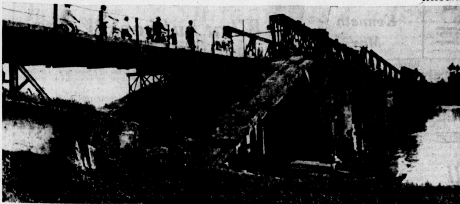
SOMETHING OLD, SOMETHING NEW — Vietnam recently. The area was heavily bombed during the Vietnam War, and this bridge, like many others, was speedily reconstructed by using the ruins of the old bridge as a base for the new one. (AP Laserphoto)
