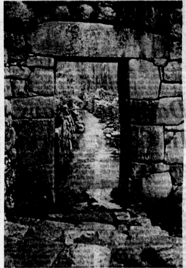
BUILT TO LAST — The stone work was rough and irregular for structures of minor importance, while temples and palaces received skilled craftsmanship. Many of the stones weighed several tons, but the Incas never devised the wheel for locomotion. (Staff Photo)
