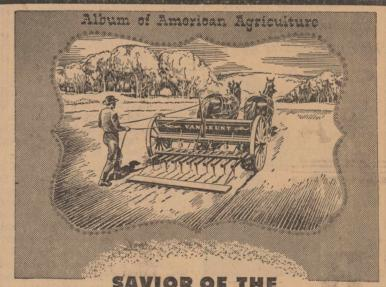
CWARMS of passenger pigeons ravaged early Wisconsin wheat crops by devouring the newly-sown grain. Moved by the farmers' plight, the Van Brunt brothers of Horicon, in 1861, built a seeder, incorporating their newly-patented cylinder feed. Seed grain was worked into the ground and covered with a protective blanket
