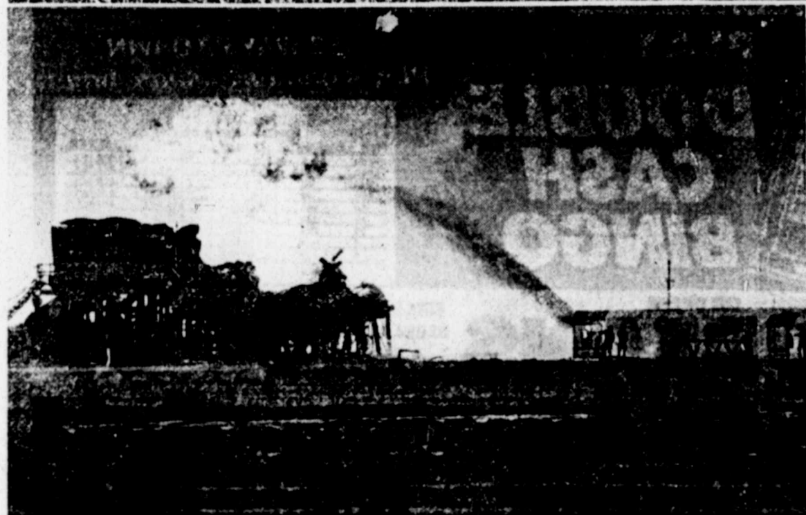
PRICE OF PROGRESS — This oilwell blowout fire, burning out of control the past five days near Loving, N.M., is gobbling up an estimated 10 million cubic feet of natural gas daily. Observers estimate the cost of burned gas at $15,000 per day. However, most of the damage was to a 162-foot derrick and platform which was destroyed when the blown out well erupted in flames early Wednesday. A-J photographer Gary Davis captured most of these fire pictures from a distance of three-quarters of a mile. The top photo shows the unattended fire raging out of control during the night, while the photo (top right) shows the scene from a slightly different perspective at day. A shielded bulldozer is visible in the photo, at right. The workmen pour a powerful stream of water onto the blaze from behind their temporary heat shields (middle photo), while others (bottom photo) drag remnants of the melted oilwell structure away from the fire. After the well area is cleared of debris, firefighters hope to blow out the fire using explosives.
