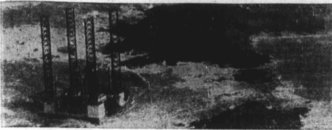
OIL RIG RUNS AGROUND — the 19,000-ton exploratory Norwegian oil rig Orion rests on rocks off the coast of Guernsey Thursday, after running aground in a force 10 gale and heavy seas during the night. The crew of the Orion—which ran aground after a towing cable parted—was being towed from Rotterdam to Brazil by the German tug Zeeveld. All the rig's crew were safely lifted off by helicopter. (AP Laserphoto)
