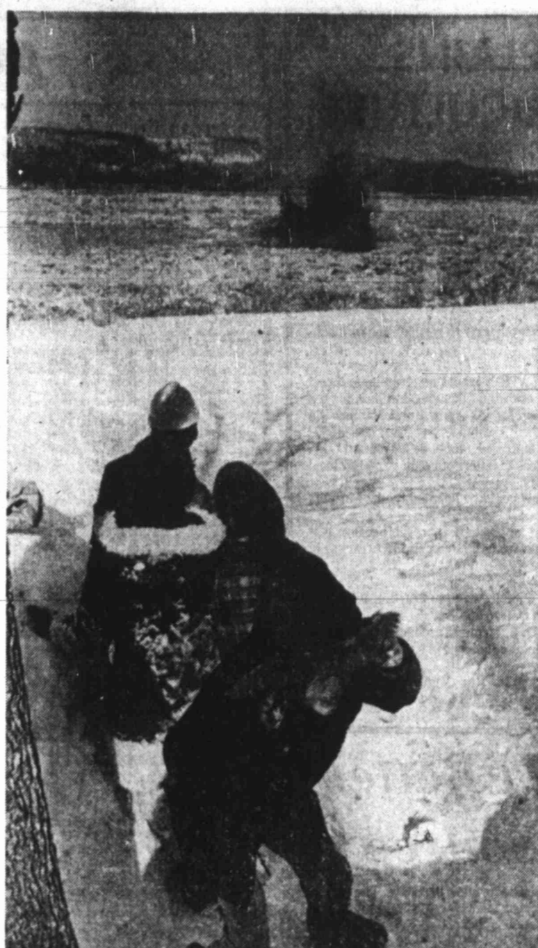
ICE BLAST—A local youngster ducks away as demolition experts blow a test explosion in the ice jam Thursday at Markland Dam on the Ohio River in Kentucky. The site is below Cincinnati. Tests using explosives with more impact broke up a section of the ice and further testing is expected today as the river ends its first week of blockage in the area. (AP Laserphoto)
