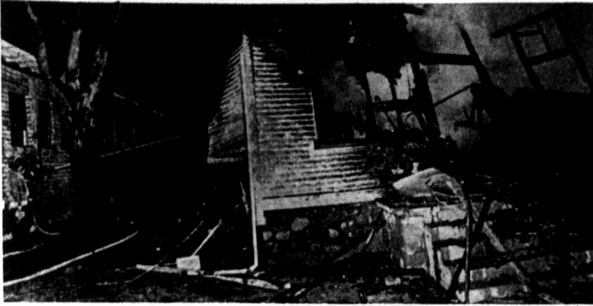
SMOLDERING INFIRMARY — Firemen Monday night hosed down the smoldering bulk of what was the Wayside Honor Ranch infirmary near Castaic, Calif., 40 miles north of Los Angeles. The infirmary was burned to the ground and at least half a dozen barracks buildings were ransacked by up to 300 farm inmates. (AP Laserphoto)
