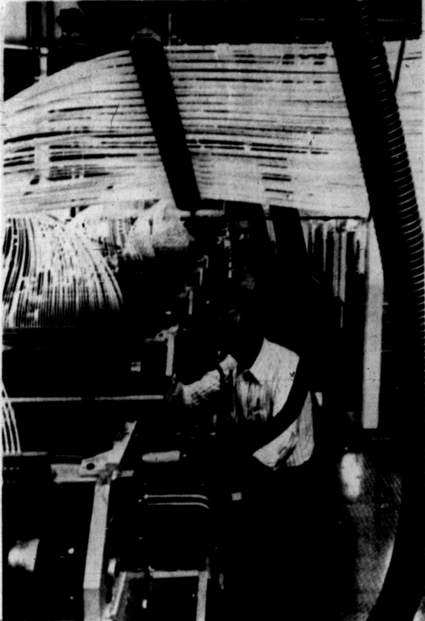
LARRY MURPHEY OF McDonnell Douglas Corp. in Huntington Beach, Calif., makes adjustments to 271-foot-long machine which will produce insulation for tanker ships that carry liquified natural gas at temperatures of minus 260 degrees recently. The machine will make a continuous log of proprietary three-dimensionally reinforced polyurethane foam. Tubes over Murphey's head feed reinforcing fiberglass into the machine. (AP Laserphoto)
