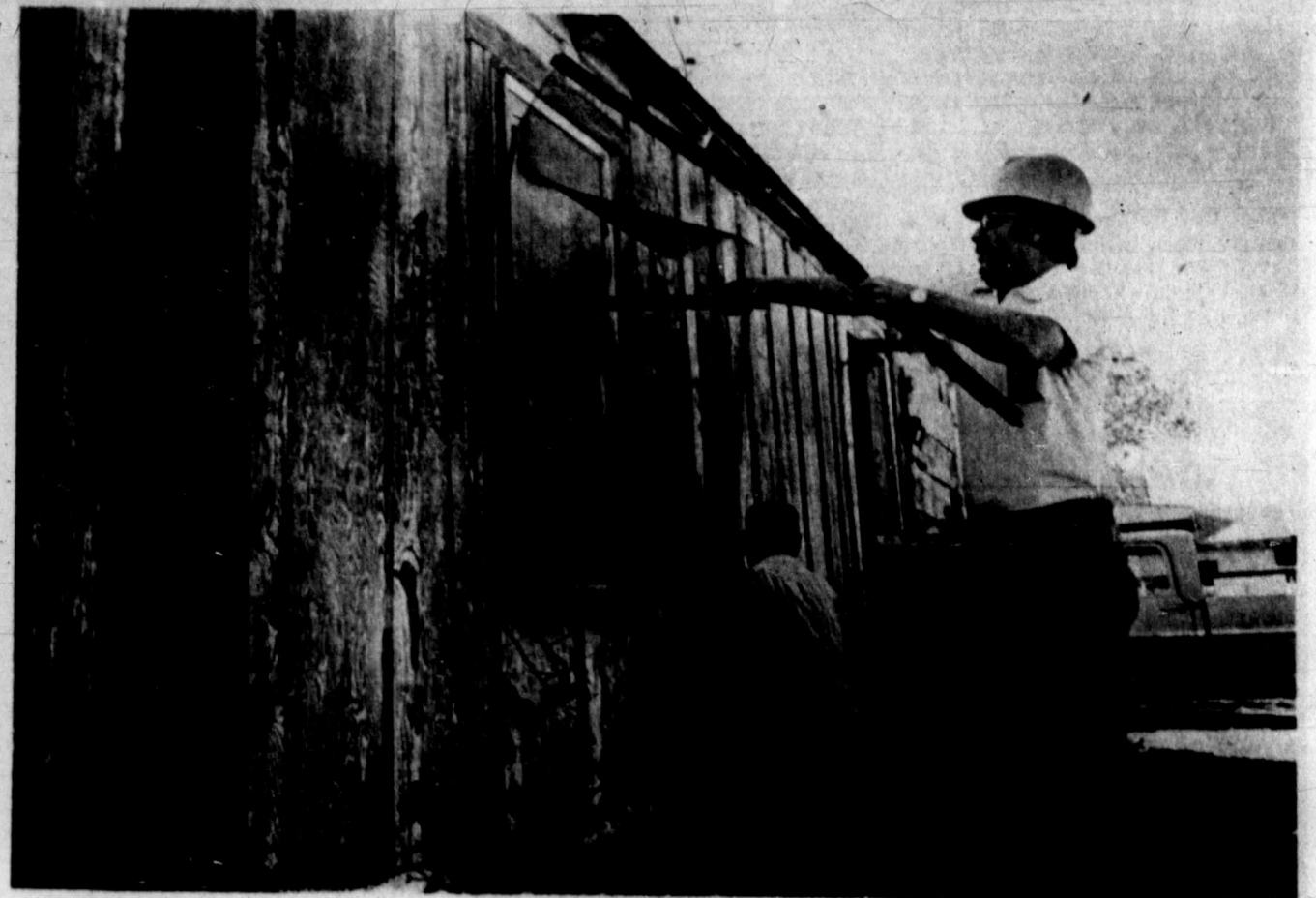
Bobby Trimble is tearing off old screens preparatory to putting on felt paper and wire.
