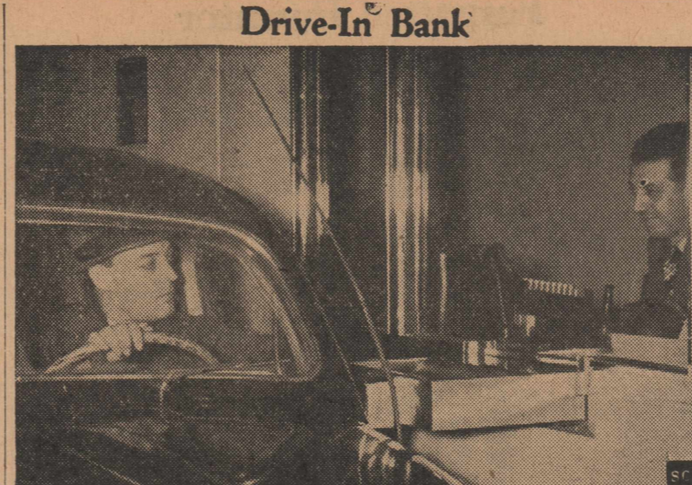
CHICAGO, ILL.—There's no parking problem for the patrons of this bank, which offers a drive-in service for its customers. As pictured above, the depositor merely drives in, takes care of his business and drives out the exit in the rear. Unusual, too, is the lack of iron bars normally associated with the teller's cage. In their place, Pittsburgh multiplate bullet-resisting glass has been used, which in addition to affording protection to bank personnel against bandits' guns, does not in any way detract from the dignity and beauty of the bank's appearance. A two-way drawer is provided at the bottom of the window for the interchange of business.
