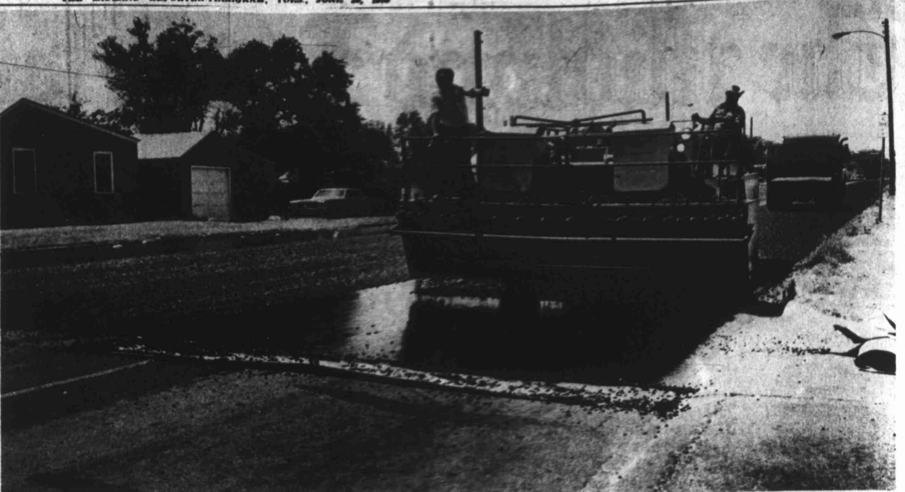
ROLLING DOWN THE gravel on North Big Spring Street are members of the city of Midland street crew, Jimmy Baldwin, left, and Alfredo Alvarado. A new layer of tar and gravel being rolled over the street is designed to give it a better surface. (Staff Photo)
