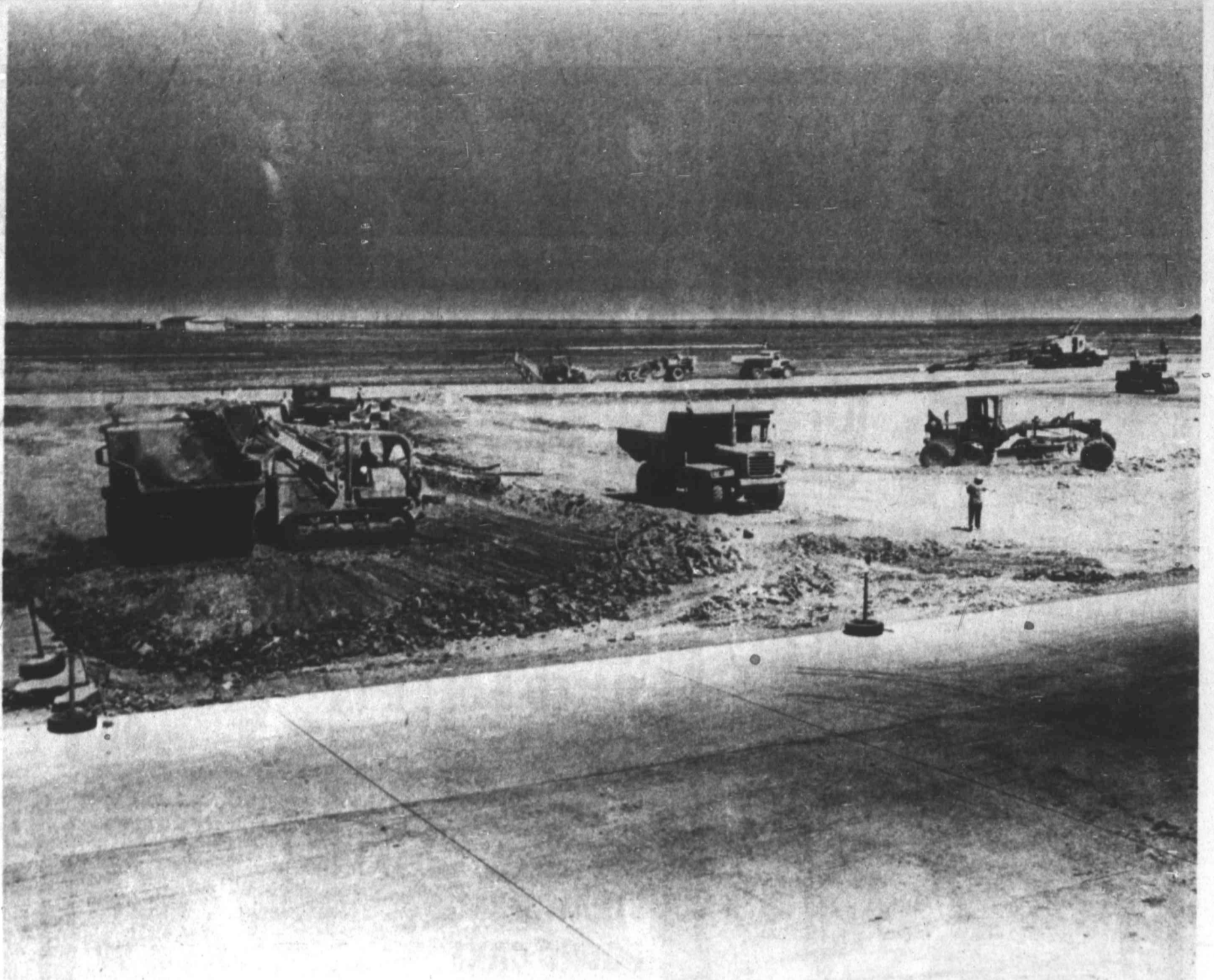
Reconstruction of runway ramps to enable larger and more aircraft to use Midland Regional Airport should be completed by November. When they were built in 1968, the Federal Aviation Administration could not foresee the tremendous increase in the number or weight of aircraft that would be using the airport.
