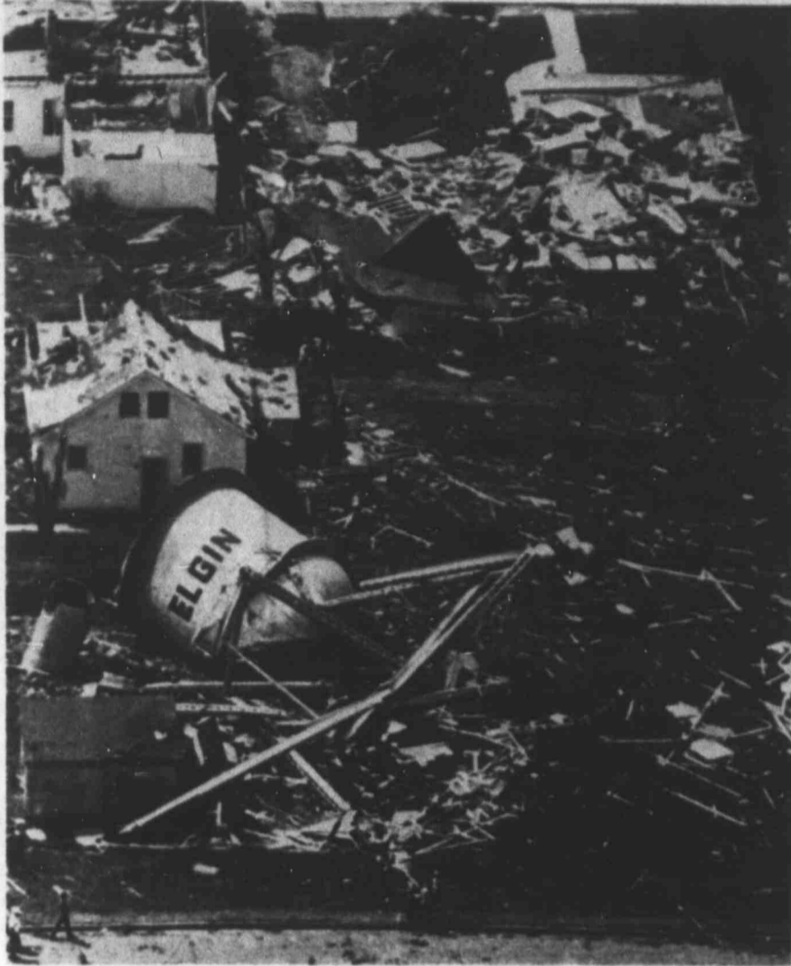
The 60,000-gallon water tower at Elgin, N.D., was demolished Tuesday night when a tornado struck the town of 1,000 people. Five were killed. (AP Laserphoto)
