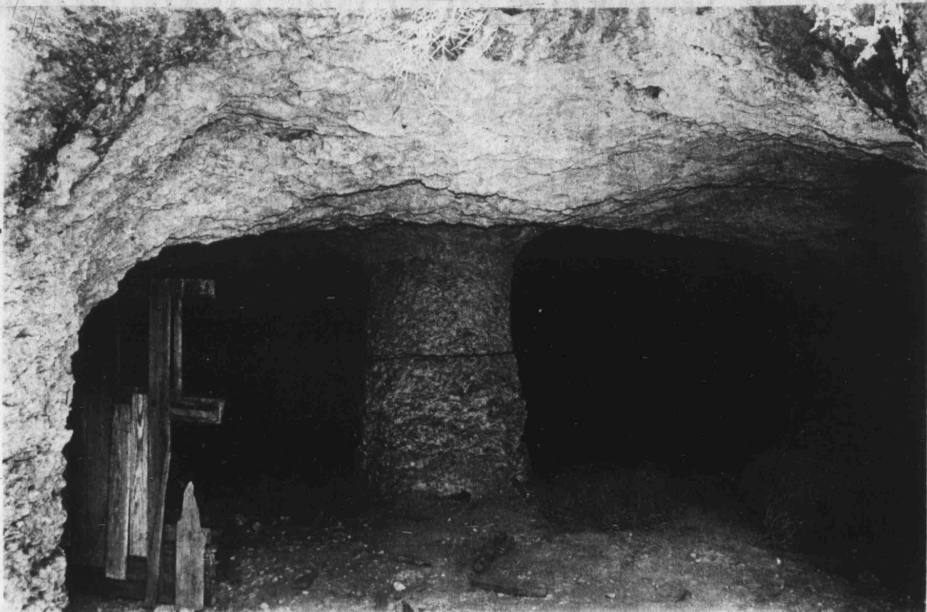
The main entrance is characterized by a large support pillar. There is room here to drive a pickup past either side of the pillar.
