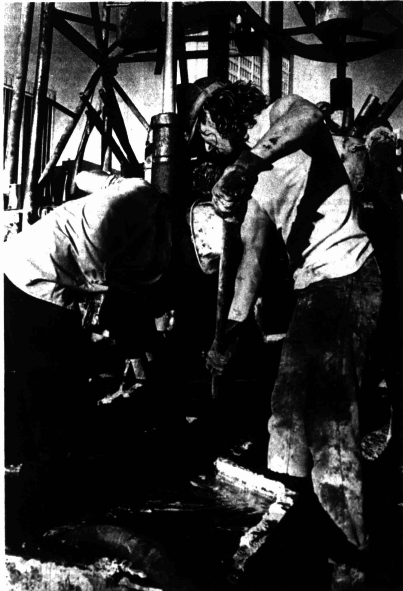
ON CLOSE INSPECTION of the background, it may appear as if oil companies have begun drilling in downtown Midland, but looks are deceiving. Actually, before construction of a building takes place, the soil must be tested to see how much
