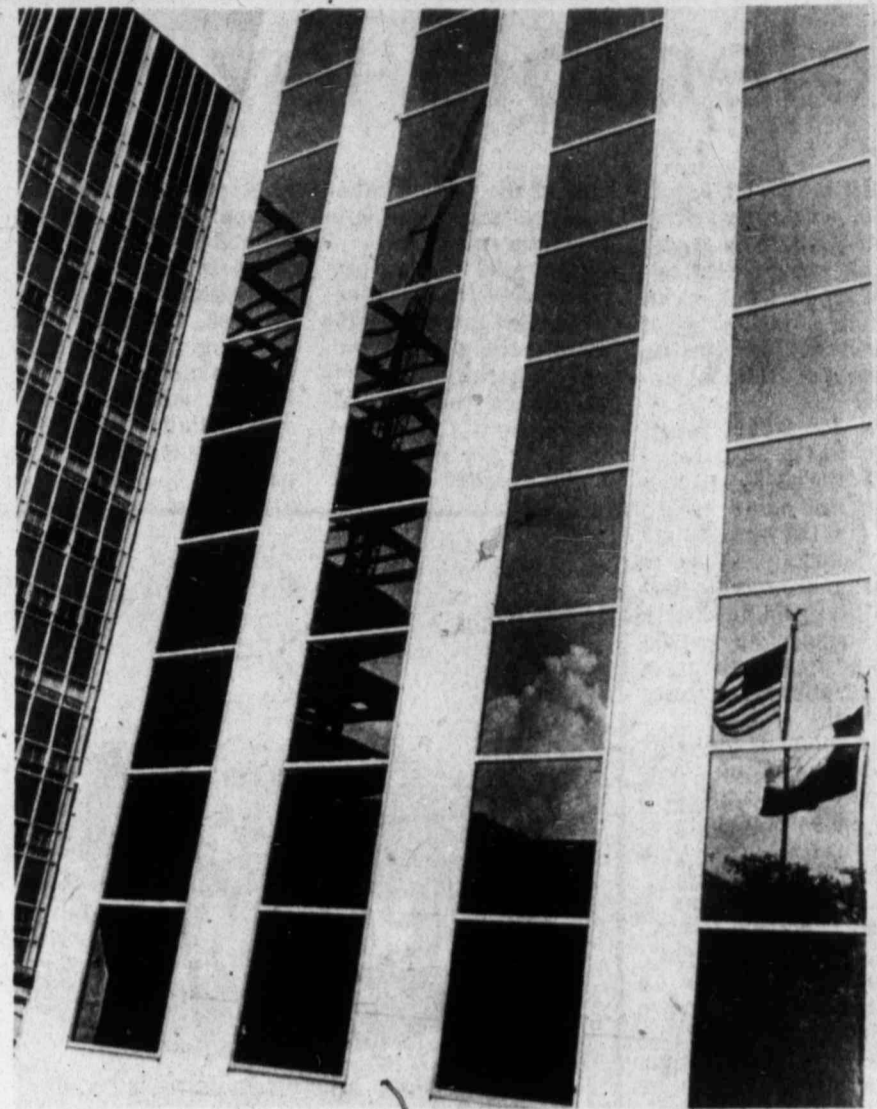
REFLECTIONS OF MORE downtown construction are seen in windows of the not-quite-completed First National Bank building as the Texas and U.S. flags wave in the background. Midland continues to improve on its nickname of the Tall City with downtown construction — mostly of the sky-challenging variety — booming these days. (Staff Photo by Mike Kardos)
