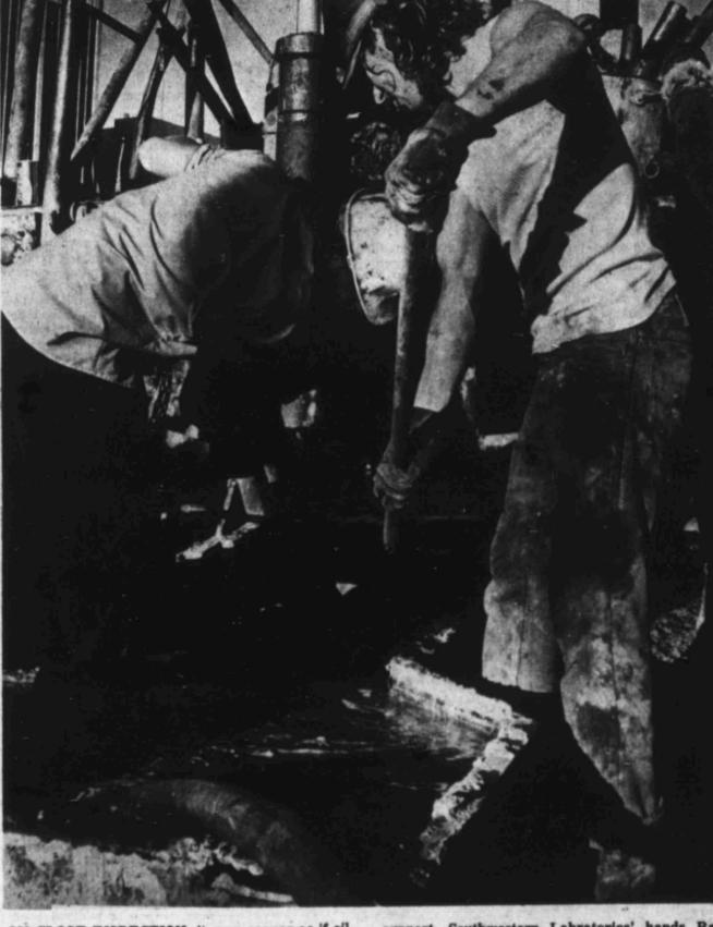
ON CLOSE INSPECTION, it may appear as if oil companies have begun drilling in downtown Midland, but looks are deceiving. Actually, before construction of a building takes place, the soil must be tested to see how much weight the area can support. Southwestern Labratories' hands Ray Kalbas, left, and Bruce Bergin work'their rig at the intersection of Lorraine and Texas streets, taking soil samples. (Staff photo by Mike Kardos)
