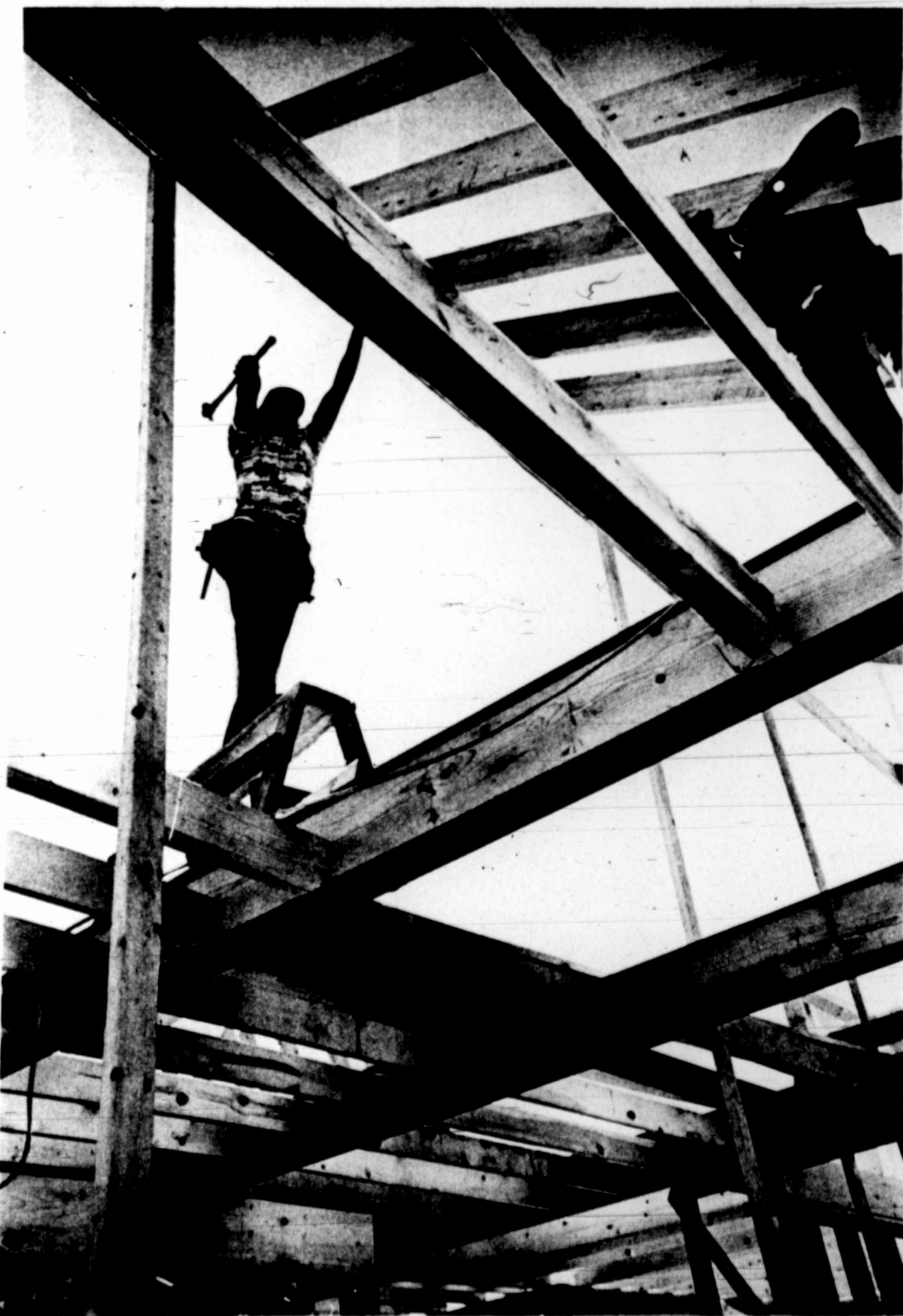
A framing crew carpenter nails in a beam at a private home in Saddle Club North addition.
