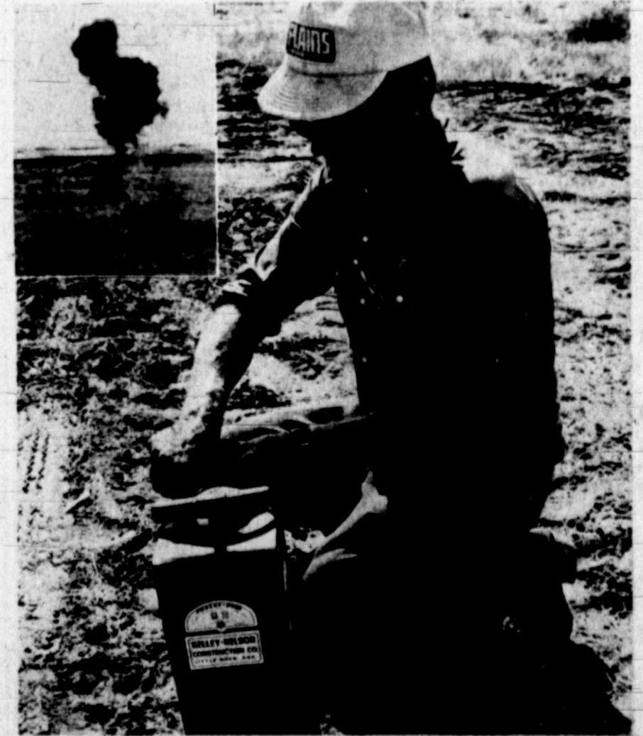
Myri Anderson of Odessa connects the detonator for one of six charges set of Tuesday in groundbreaking observances for Midland Mall. A small puff of smoke and a blast of noise resulted from each of his efforts, as intended. (Staff Photo)
