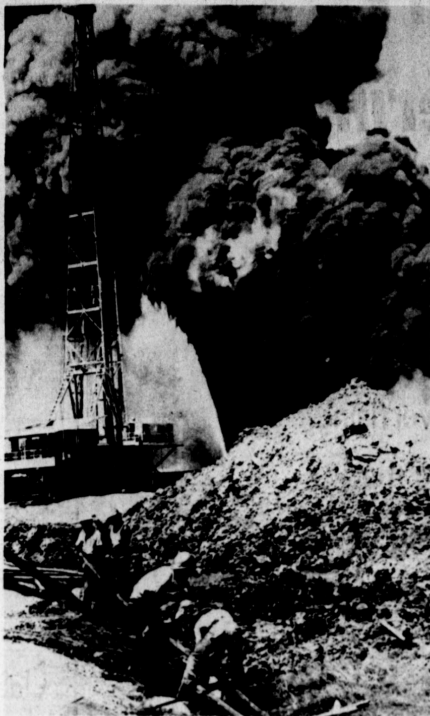
Workmen put down pipe while a fire burns at an underground oil storage facility at West Hackberry, La. The new pipeline will be used to drain out some of 7 million barrels of oil stored in the salt dome to relieve pressure and aid in putting out the blaze that erupted Thursday killing one man and seriously injuring another. (AP Laserphoto)
