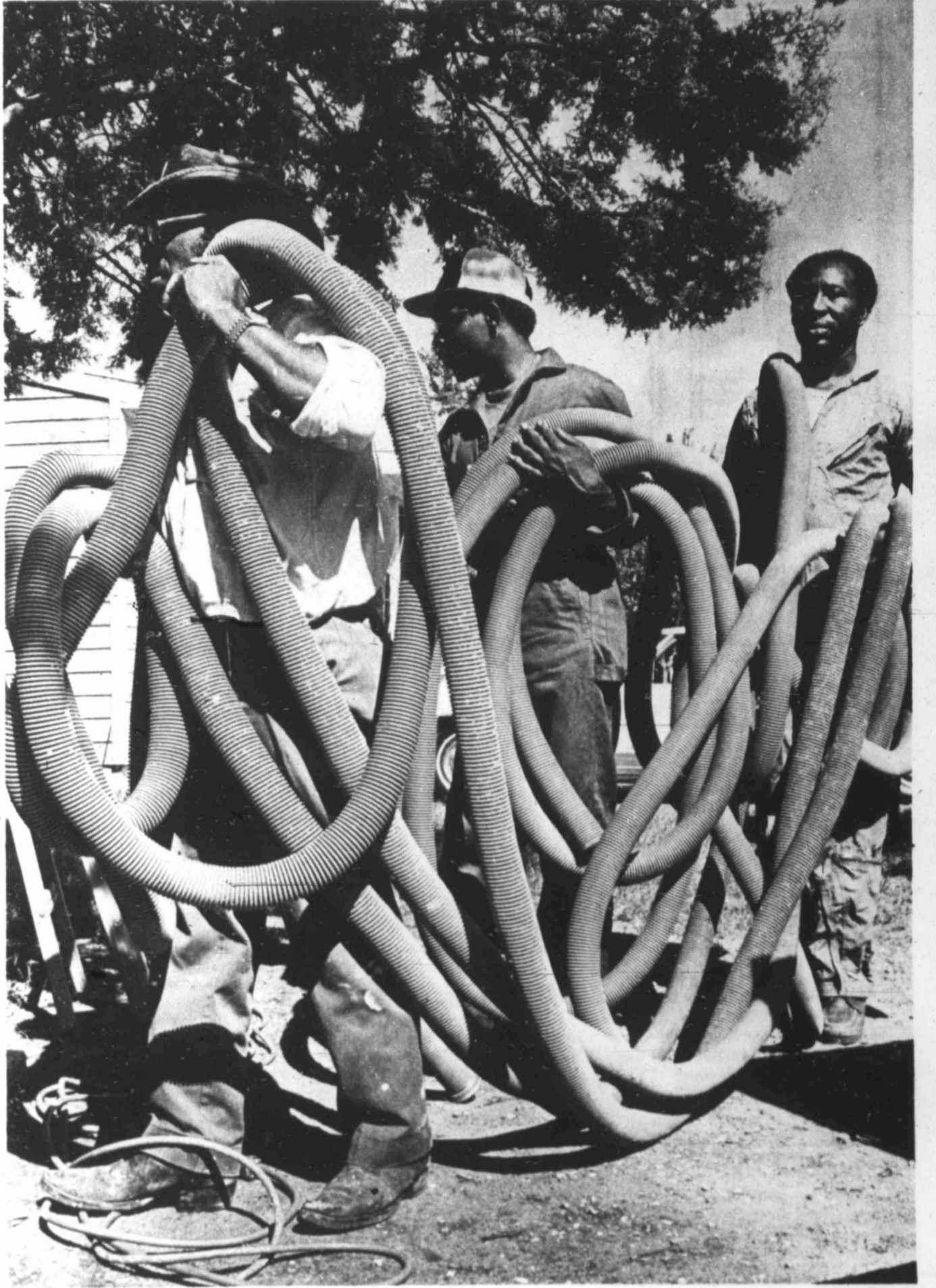
Grabbing hose to be connected to an insulation blowing machine are, from left, Earnest Jones, Anthony Foy and Albert Jones, weatherization coordinator for the Midland County Community
