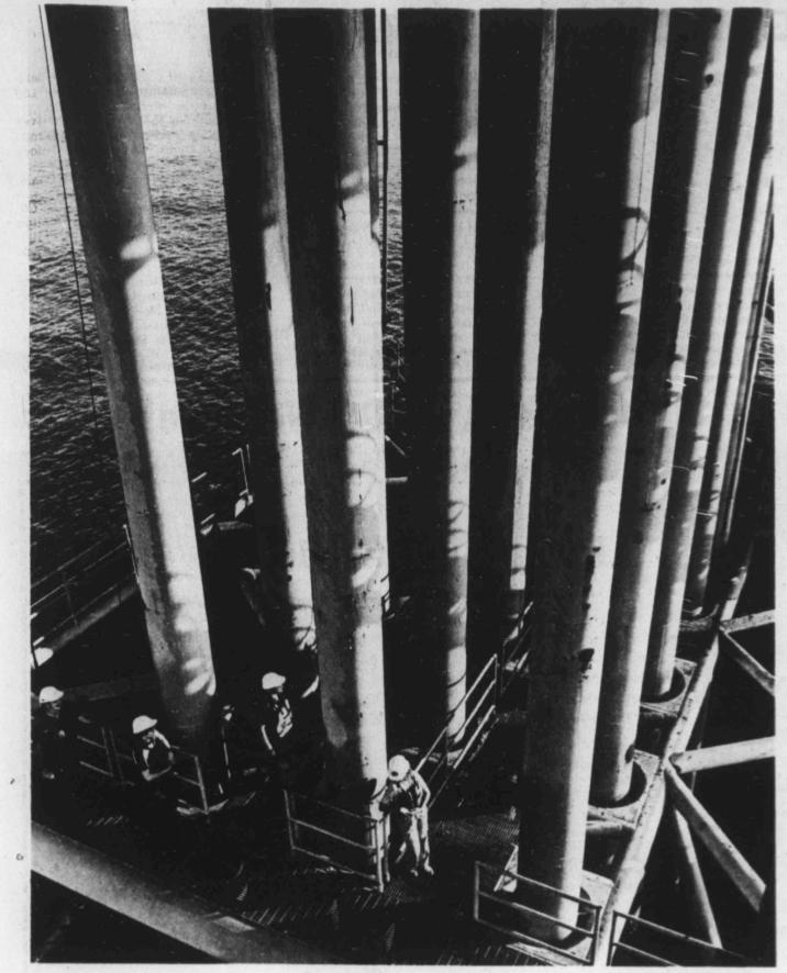
Like columns of an ancient temple, steel jackets abound beneath a Tenneco Oil Co. platform in the West Cameron area of the Gulf of Mexico. Driven into the Gulf floor, they extend high above the
